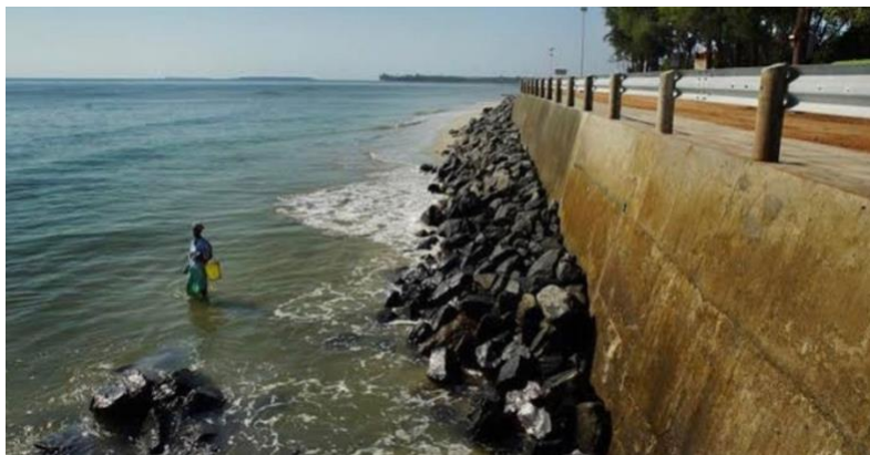
Image 3; a 780m sea wall at Barack Obama road constructed by the Government of Tanzania as a response to effects of climate change.
