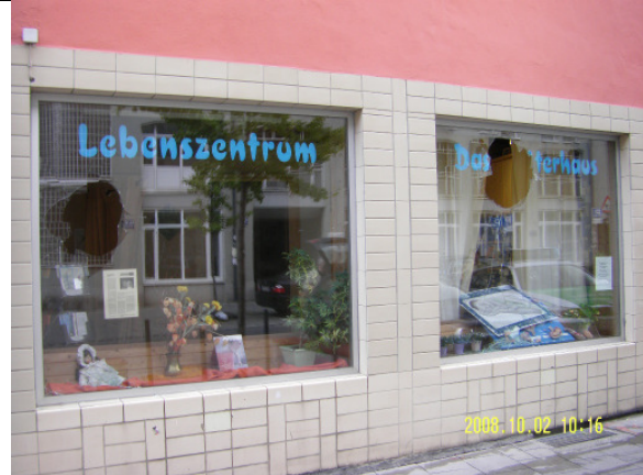
The damaged windows of the Munich Life-Center
